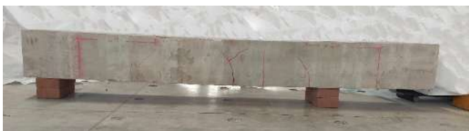
Figure 16 Crack pattern at failure for precast specimen AAC 25x25-1.
