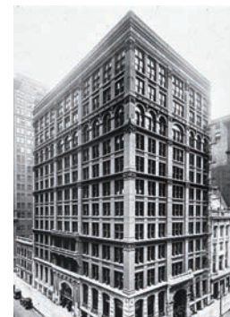
HOME INSURANCE BUILDING CHICAGO, 1885
