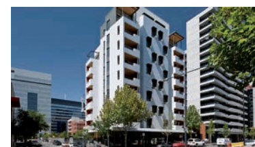
FORTÉ BUILDING IN MELBOURNE, AUSTRALIA. PROGETTO LEND LEASE.
