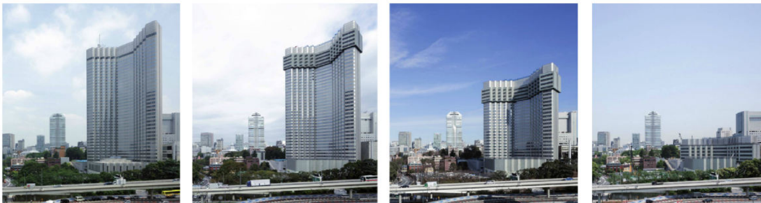
Tecorep System applicato al Grand Prince Hotel Akasaka (per cortesia Taisei)
